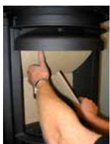
4. Once the side brick and the rear brick panels have been removed, lower the bottom baffle and lift it out.
